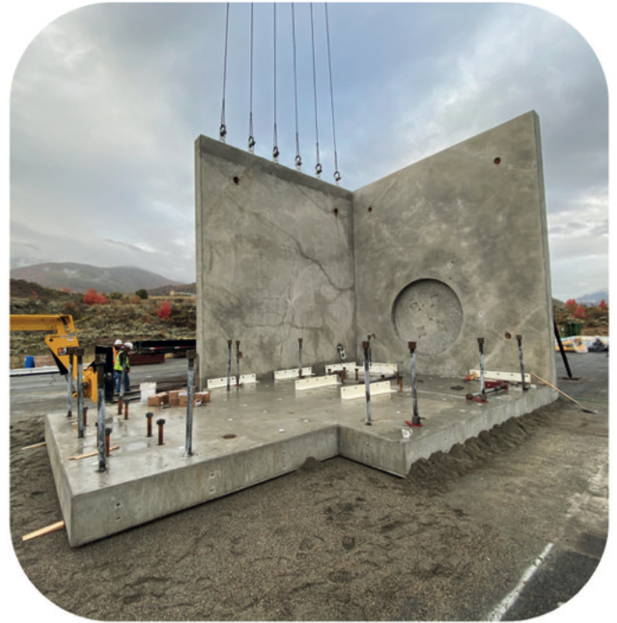
New Bypass Exit Portal being dry fit prior to underwater placement
