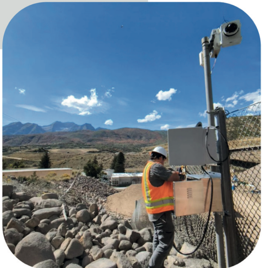
Upgrading wireless radio installation
