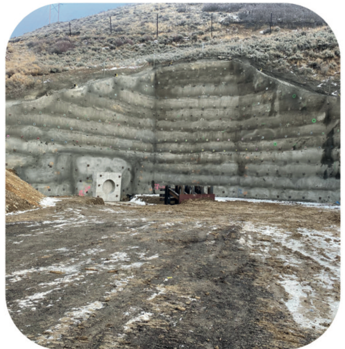
Soil nail wall and MTBM launch portal headwall and thrust restraint
