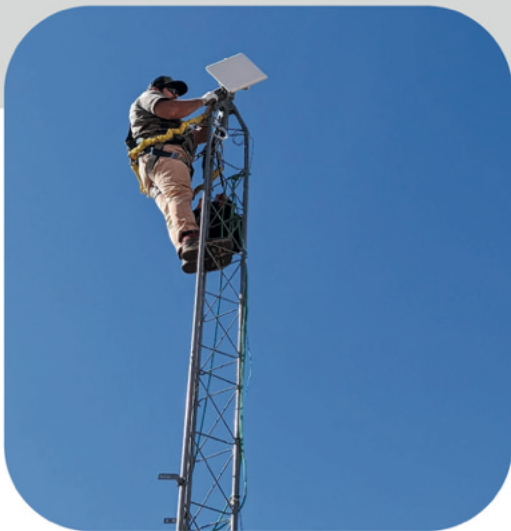
Upgrading wireless radio installation
