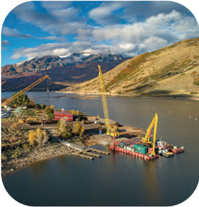
Sailboat Beach construction and staging area
